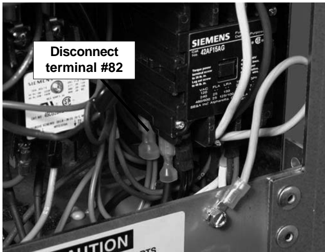
Figure 5-2 Disconnect Compressor Coil
