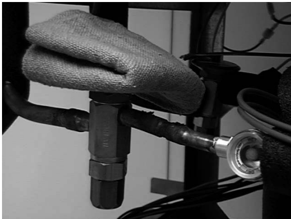
Figure 5-5 AXV Removal
