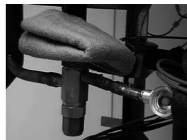
Figure 5-4 TXV Removal
