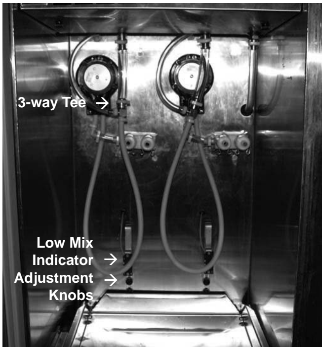
Figure 2-6 Connecting Pump Hose to BCS Manifold
