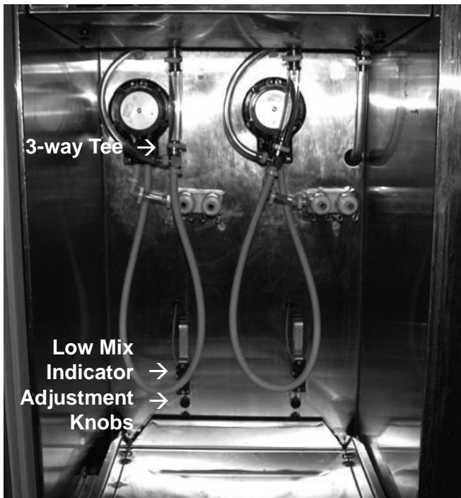
Figure 2-6 Connecting Pump Hose to BCS Manifold
