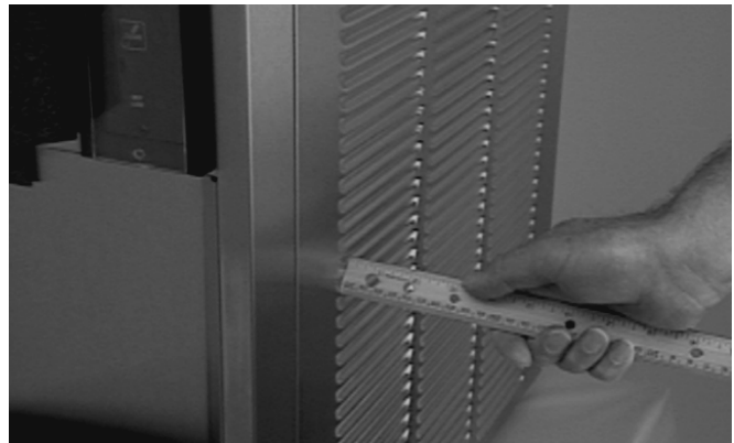
Figure 5. Space and Ventilation Requirements
