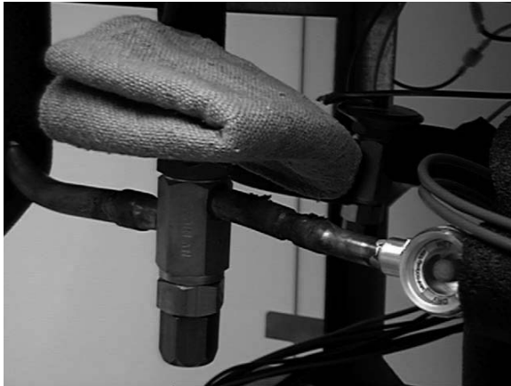
Figure 5-5 TXV Removal
