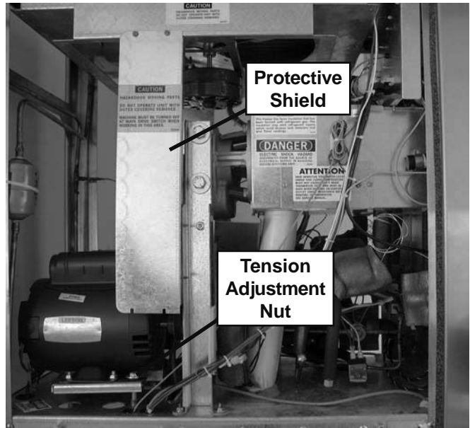
Figure 6-5 Motor Removal
