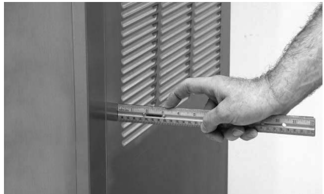
Figure 2-1 Space and Ventilation Requirements
