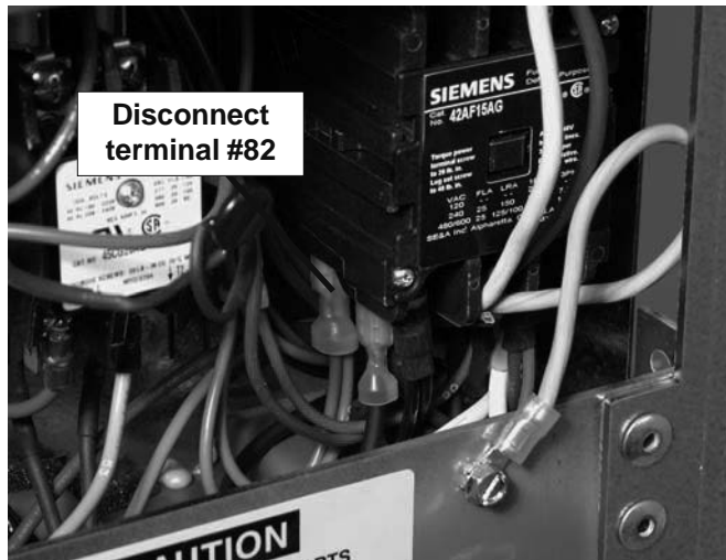
Figure 5-2 Disconnect Compressor Coil
