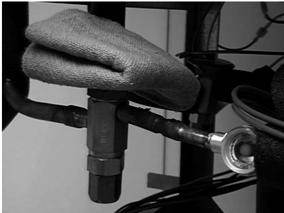
Figure 5-5 TXV Removal
