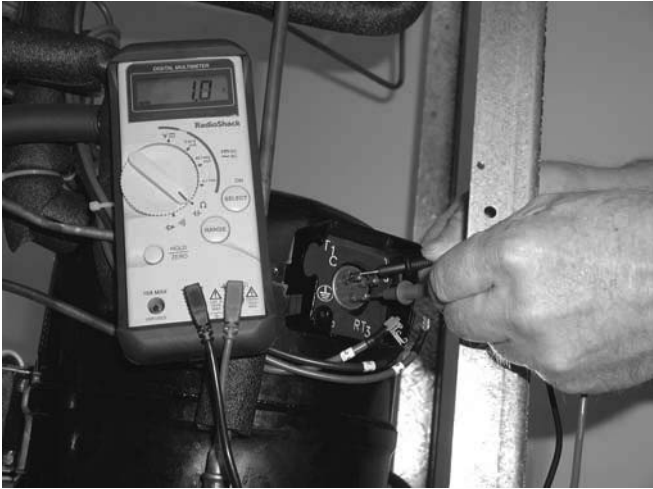
Figure 13. Ohm Meter Connection
