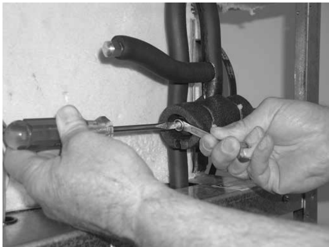
Figure 20. EPR Valve Adjustment
