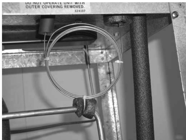
Figure 23. Drier Cap. Tube Assembly
