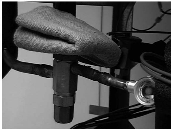
Figure 5-5 TXV Removal
