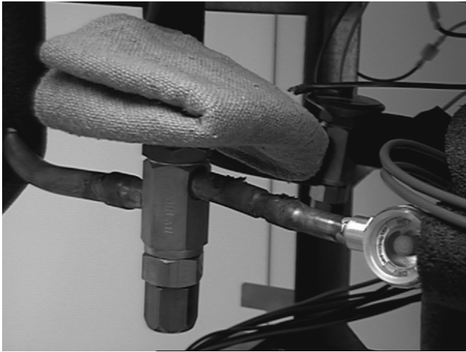
Figure 42. Expansion Valve Removal
