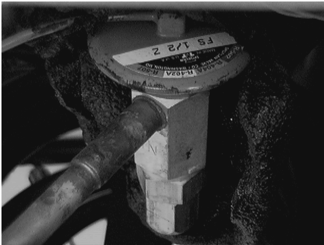
Figure 41. Expansion Valve
