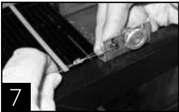
Door roller bracket with metal cable.
