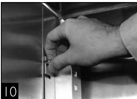
Pilaster installation (side wall of cabinet)
