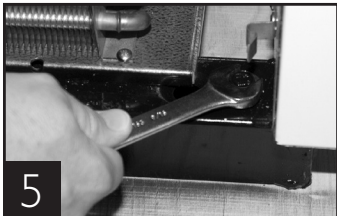
Images 4-6, removing skid from bottom of cabinet.
