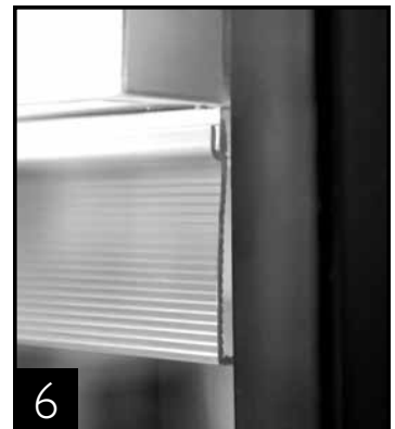
6 lampshield "U" channel in position over metal bracket.
