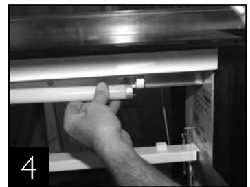
4 Remove bulb by gently pushing bulb into spring loaded lampholder.
