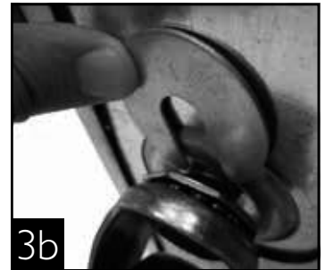
Installing castors (shims)
