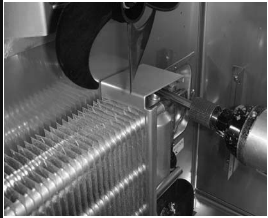
A.Remove the evaporator coil
