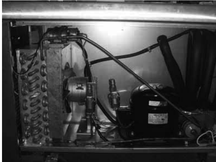
CONDENSING UNIT ASSEMBLY TCBE-52SDR
