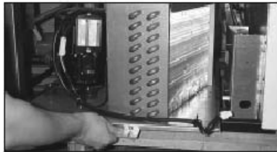
4. Pull the Compressor Base and separate the Condenser Fan Motor.
