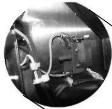
High Limit Switch Reset Button
